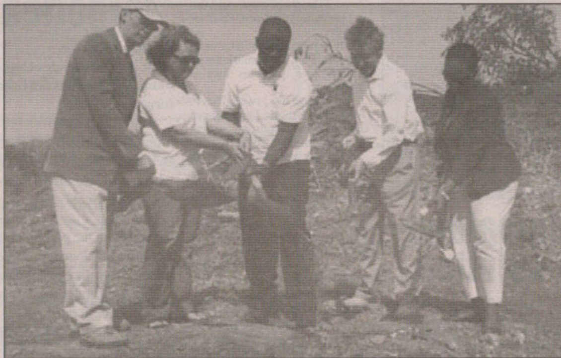
The first shovels hit soil as work on the new youth centre begins.
